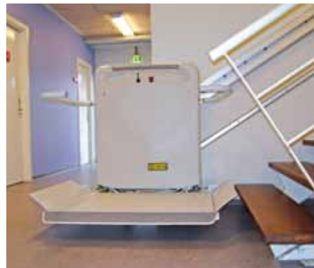
Indoor installation with a walk through hall limiting free space down stairs. After use lift will be folded up and run up the stairs to be parked away.
