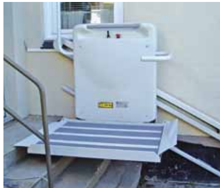
Outdoor installation on wall. Private house, Denmark.
