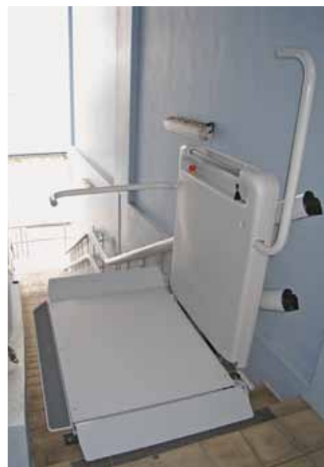
Outdoor installation bend over horizontal landing. Singapore, Malaysia.
