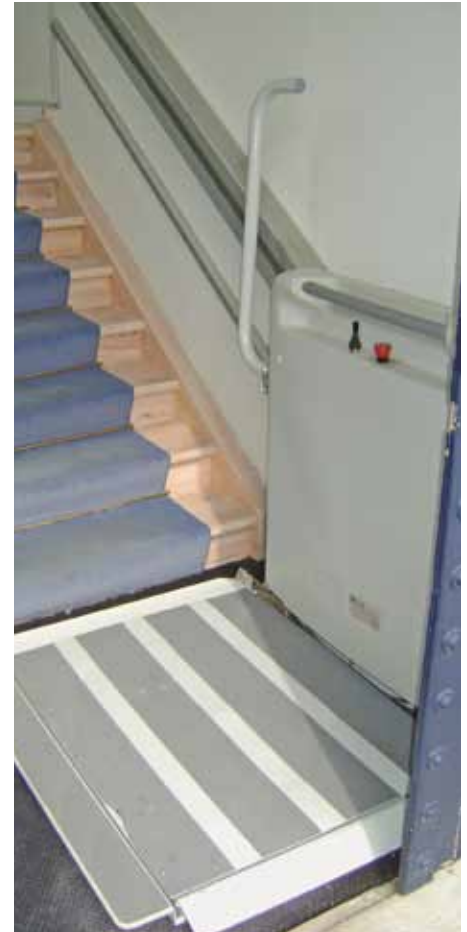
Entrance to the lift with a side access on the platform
