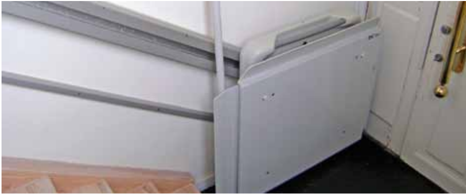
Indoor installation parked and folded lift, limited space down stairs.
