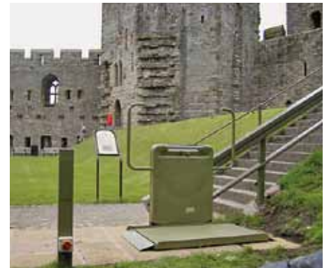
Outdoor installation on stanchions. Slides down slope next to stairs. Castle, UK.
