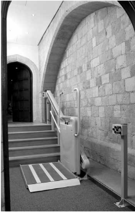
Indoor installation on stanchions. Palace of Westminster, UK.
