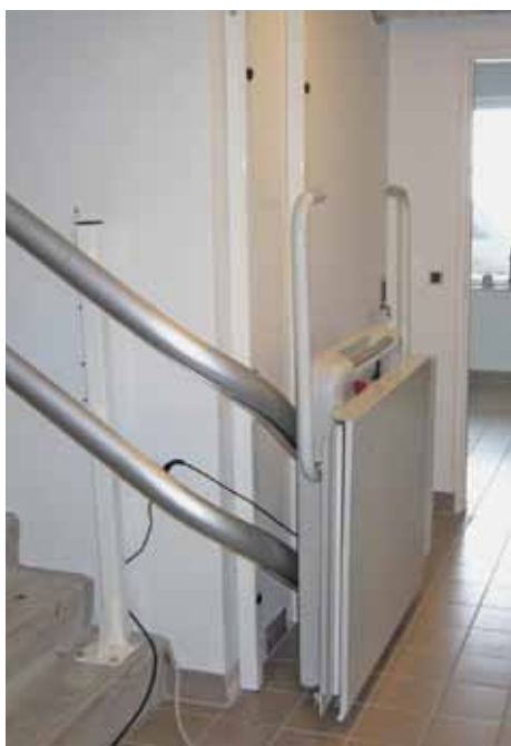
Indoor installation 180° bend down stairs.
